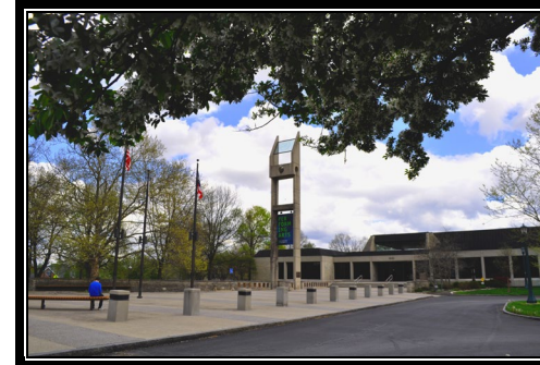
Municipal Services Center
