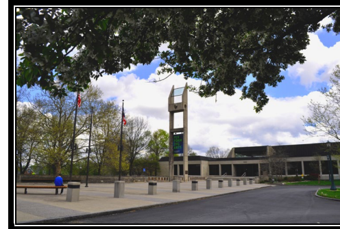
Municipal Services Center
