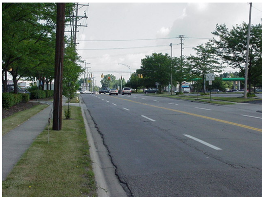
Reed Road Looking North Near Henderson Road
