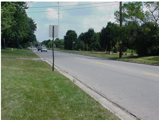
North Star Road Looking North Near Northwest Boulevard
