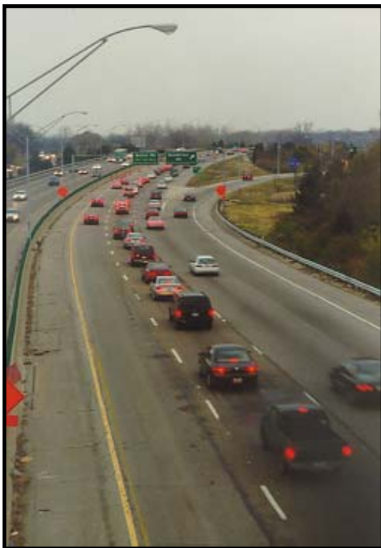
SR 315 Near Henderson Road
