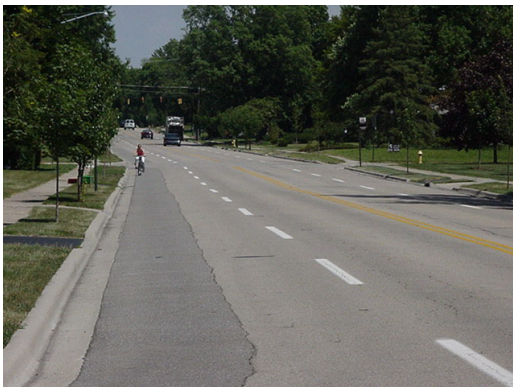
Zollinger Road Looking East at Avalon Road
