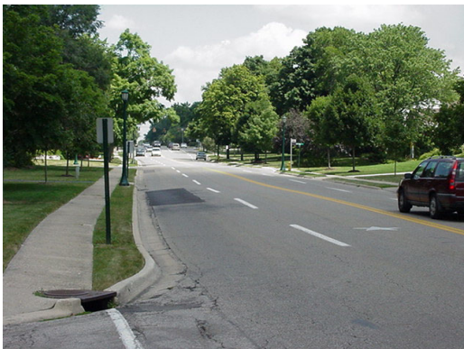
Northwest Boulevard Looking North Near Chatfield Lane
