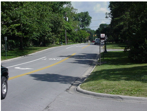
Tremont Road Looking North Toward Lane Avenue
