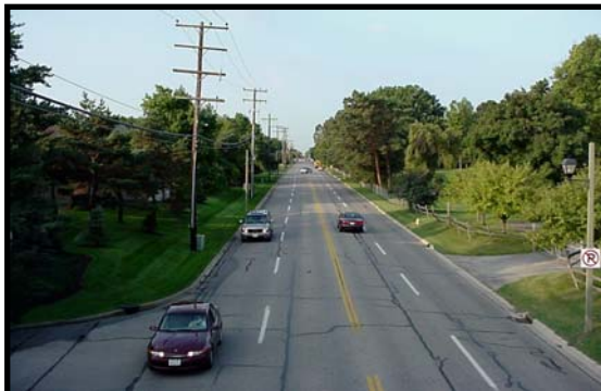
Tremont Road – Typical Upper Arlington Four-Lane Undivided Corridor with 10-to 11-foot Lanes
