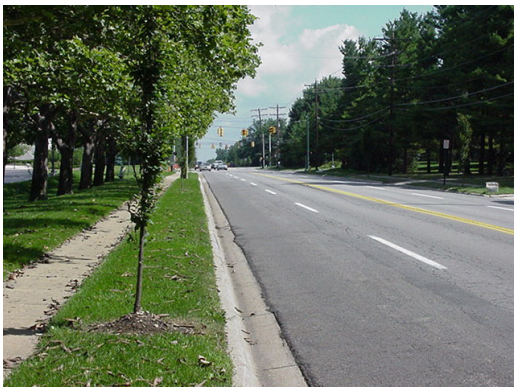
Reed Road Looking North Near McCoy Road
