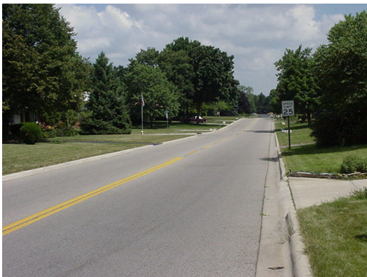
North Star Road Looking North Near Zollinger Road
