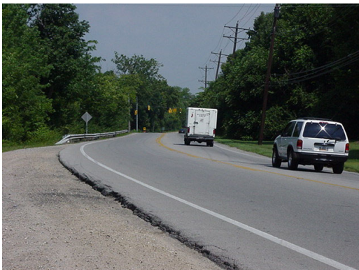
Riverside Drive Looking North Toward Henderson Road
