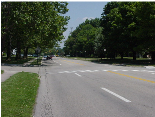
Zollinger Road Looking East Toward Northwest Boulevard
