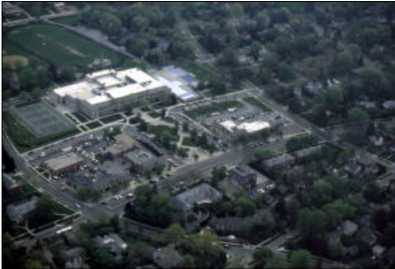
Mallway looking northwest
