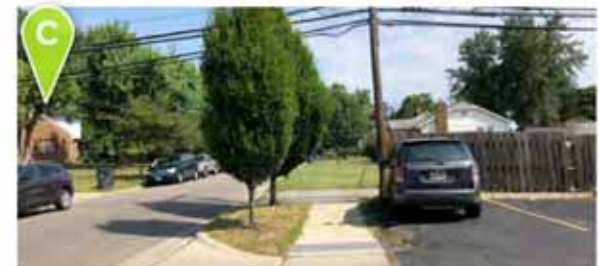
Missing sidewalk entering the corridor from neighborhood.
