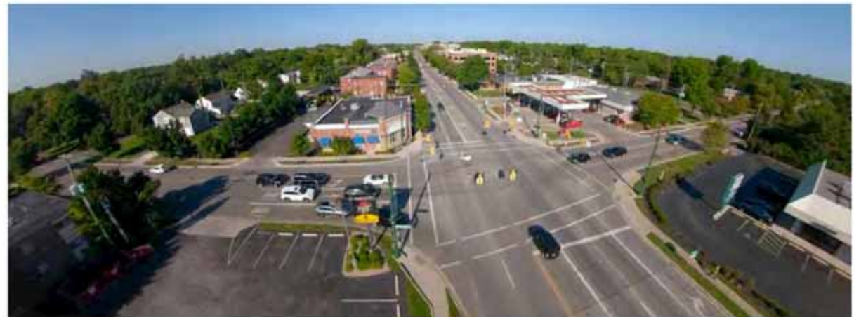
FIGURE 25: Existing Condition Looking West on Lane Avenue
