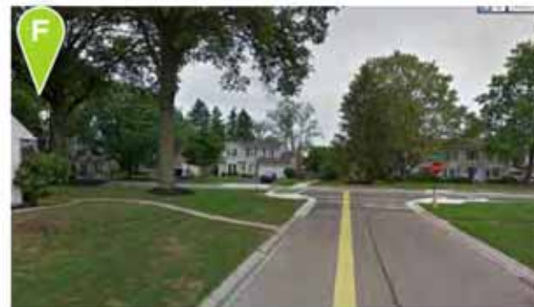
Missing sidewalk entering the corridor from neighborhood.
