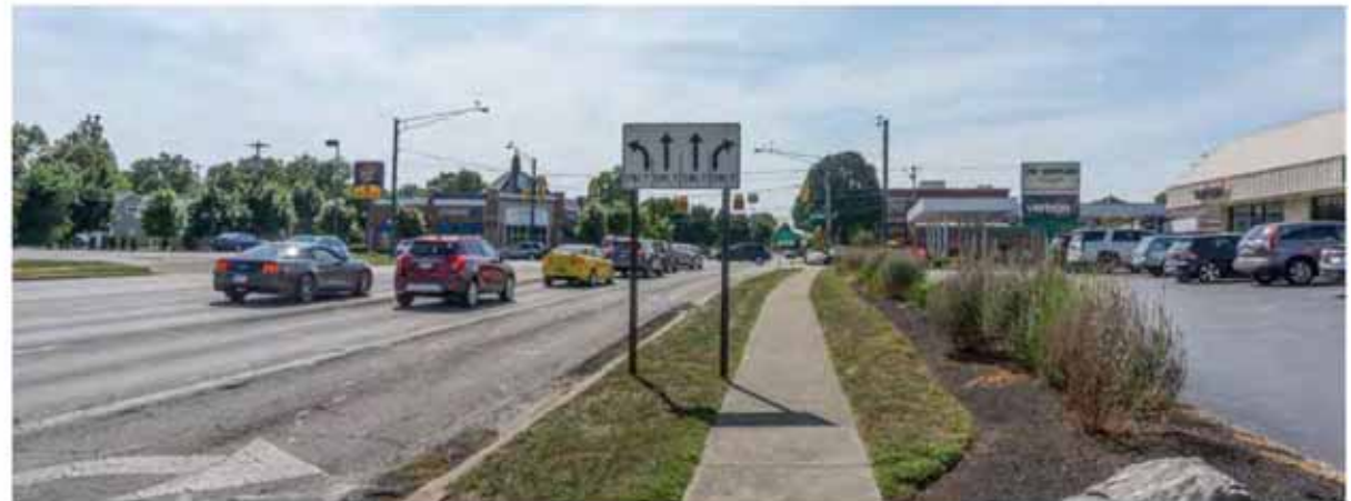
FIGURE 9: Existing Condition near North Star Road, Looking West
