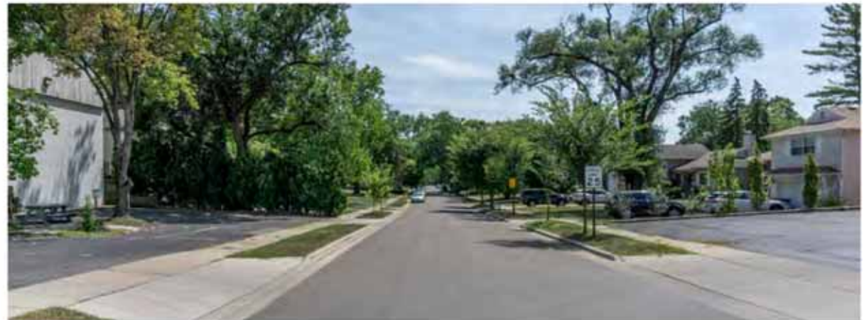
FIGURE 15: Existing Condition at Brandon Road, Looking South
