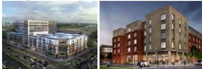
Figure 4: Arlington Gateway (left) and Lane II (right) are anticipated to add a total of 150,000 sf of office space.
