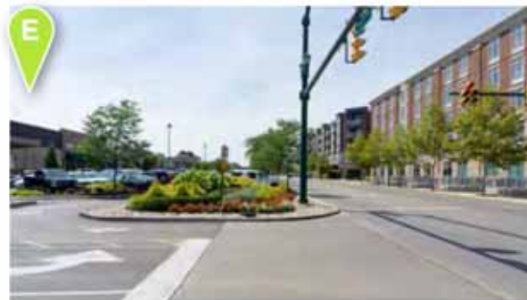
Missing sidewalk in front of Shops on Lane Avenue.
