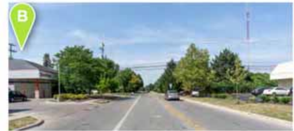
Missing sidewalk on east side of North Star Road.
