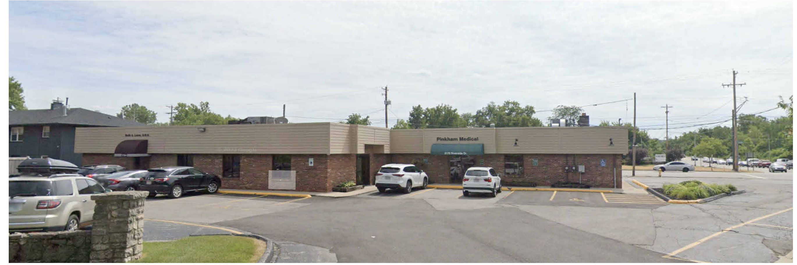
EXISTING VIEW OF EAST ELEVATION
