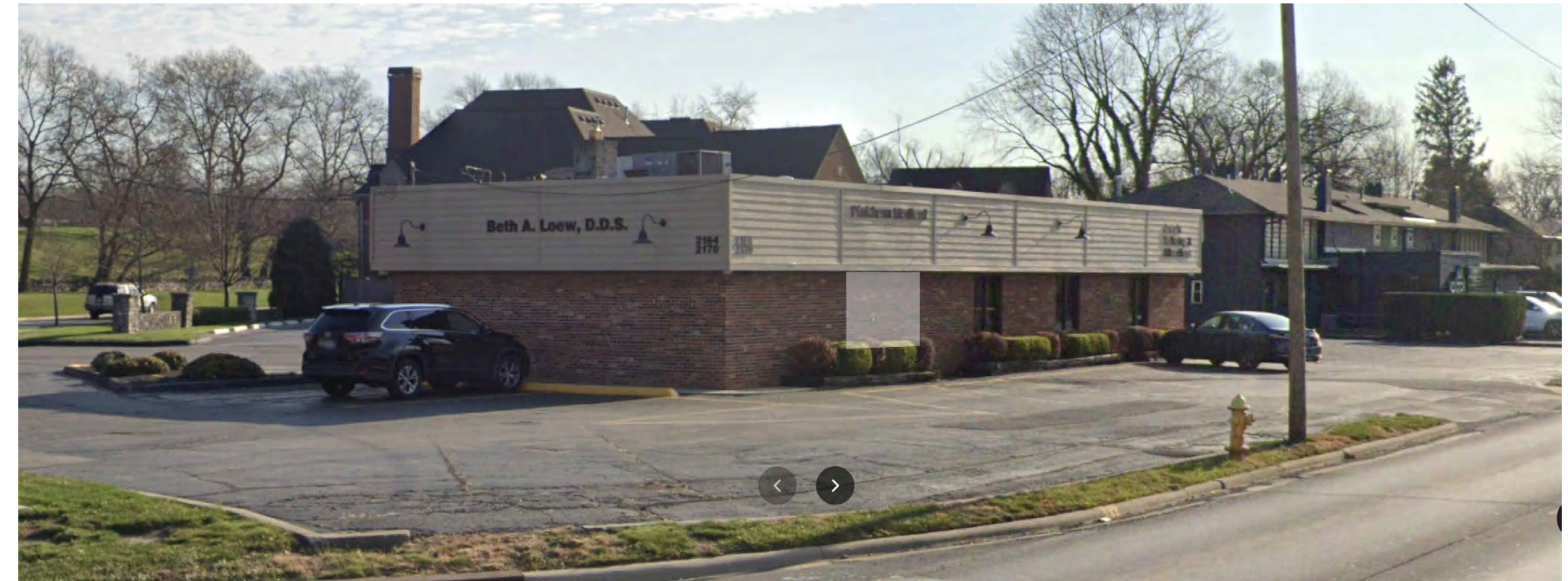
EXISTING VIEW OF NORTHWEST CORNER
