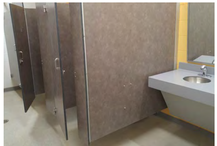
New bathrooms at the pool concession building
