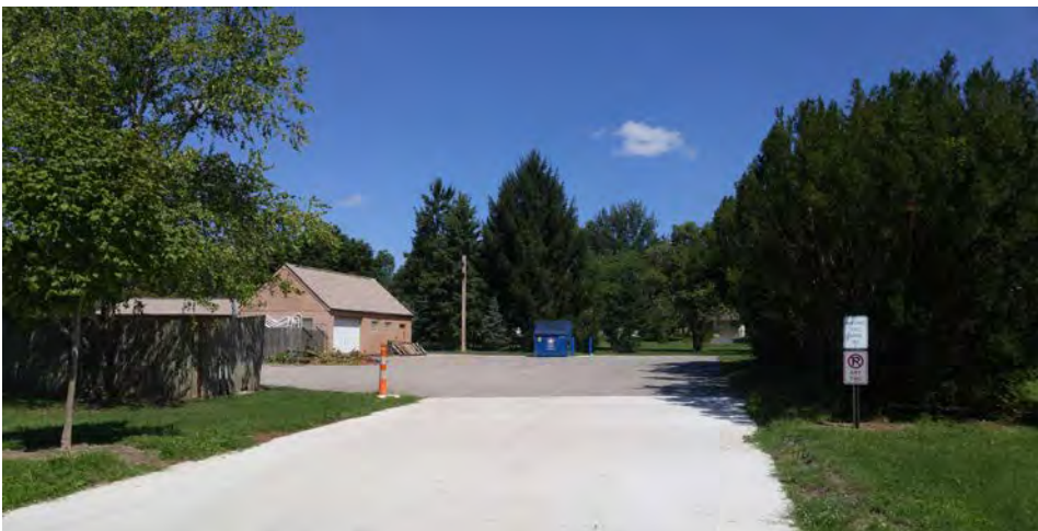
Facilities building entrance
