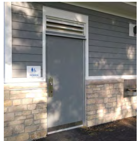
New bathrooms at the pool concession building
