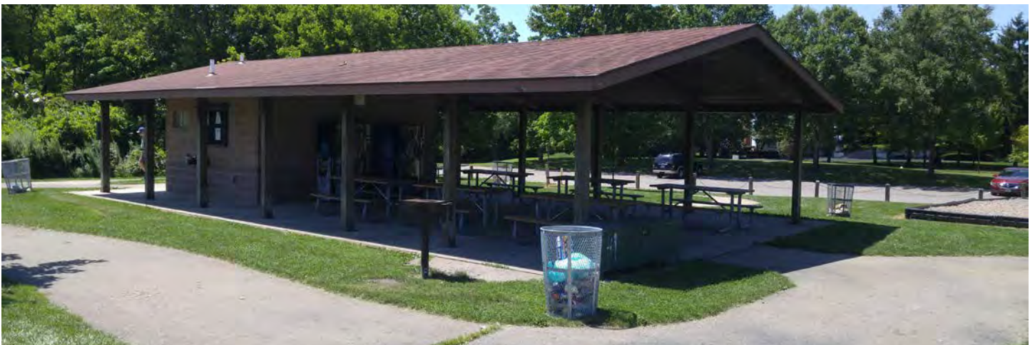
Shelter building with picnic area, restrooms, grill, and drinking fountain
